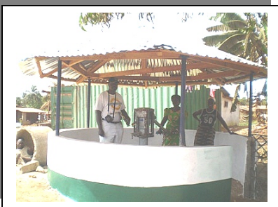
Top - finishes well Right- worker going down in well
